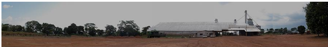
Figure 3. Grain drier in Fabio's hometown. The dryer started operating in 2017 and is owned by landholders who are transitioning into capital-intensive soy farming.
